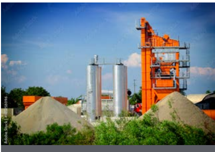
Asphalt mixing plants
